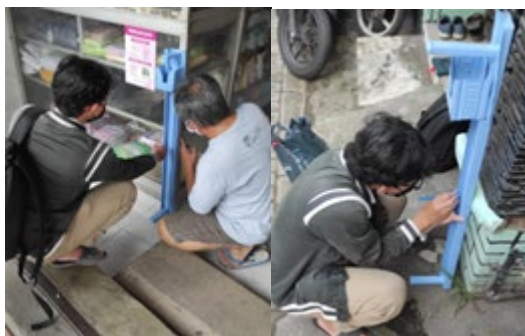
Gambar 3. Pemasangan hand sanitizer pedal
